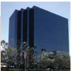
611 ANTON - BUILDING I
