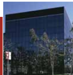
675 ANTON - BUILDING III
